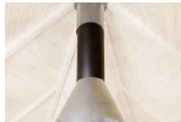
Grill Chimney Extension
